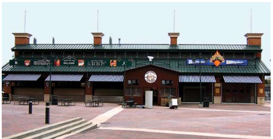
Skip & Pete's Rinnai installation resulted in reclaiming about 40 square feet of floor space after removal of a 200-gallon water tank and a 650,000-BTU boiler.
